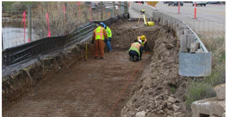
Crews begin work on a retaining wall on the north side of the Flat Creek Bridge.
