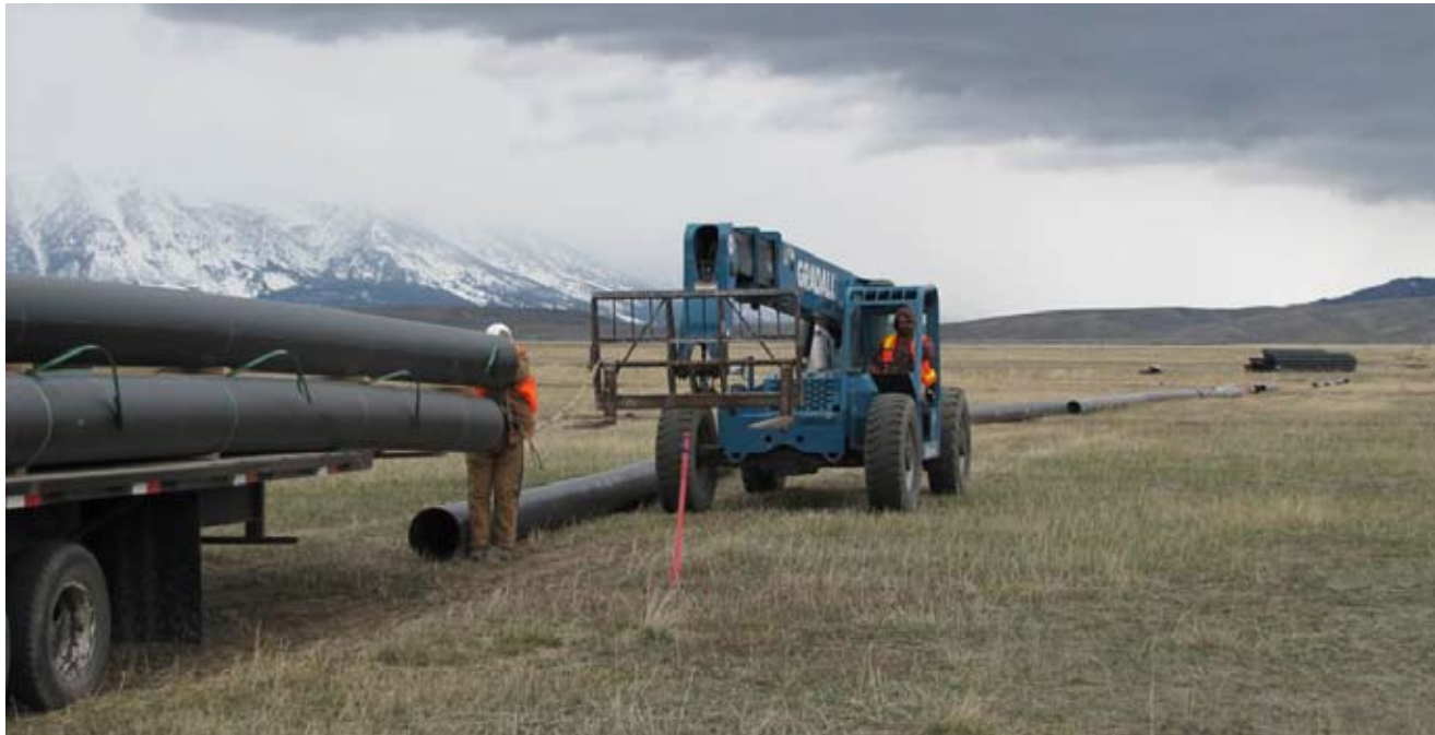
Crews lay pipe in place in preparation for fusing and installation.
