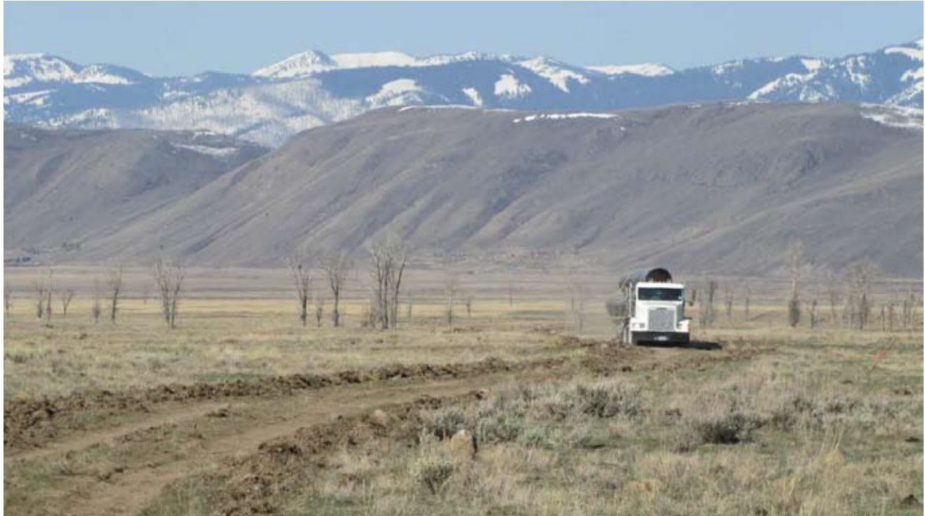
A semi truck hauls irrigation pipe from the delivery site to a staging area closer to the head of the project near Flat Creek. Trucks are using a temporary road cut in to accommodate the large vehicle traffic. The road follows the basic route that will be excavated for pipeline installation, minimizing disturbance and the need for additional restoration.
