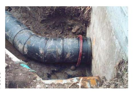
A new section of 24" diameter pipeline (top) is fastened to the concrete headgate next to an existing 27" pipeline (bottom). Water from Flat Creek was temporarily diverted during the operation.
