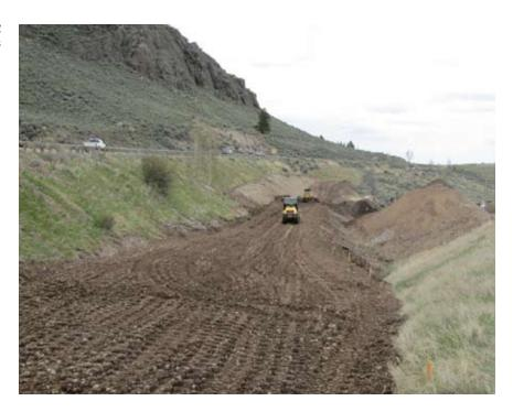
restriction that pathway grades must be limited to less than a 5% longitudinal slope, making them compliant with American Disabilities Act (ADA) guidelines. Without the side hill work, the pathway would present an approximate 10% grade increase, a steep gain that would not fit within the scope of the project.
